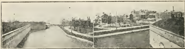
MOAT. FT. MONROE. FROM THE RAMPARTS.
